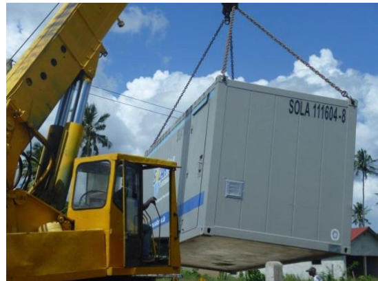
A special crane lifted the container off the truck....
