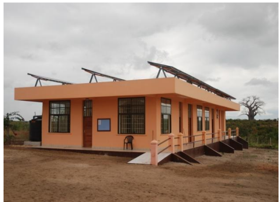
Installed Solar Panels
