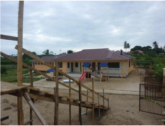
A provisional ramp was set up to facilitate the transport.....
