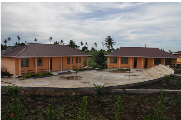
The new school amphitheatre has been completed.
